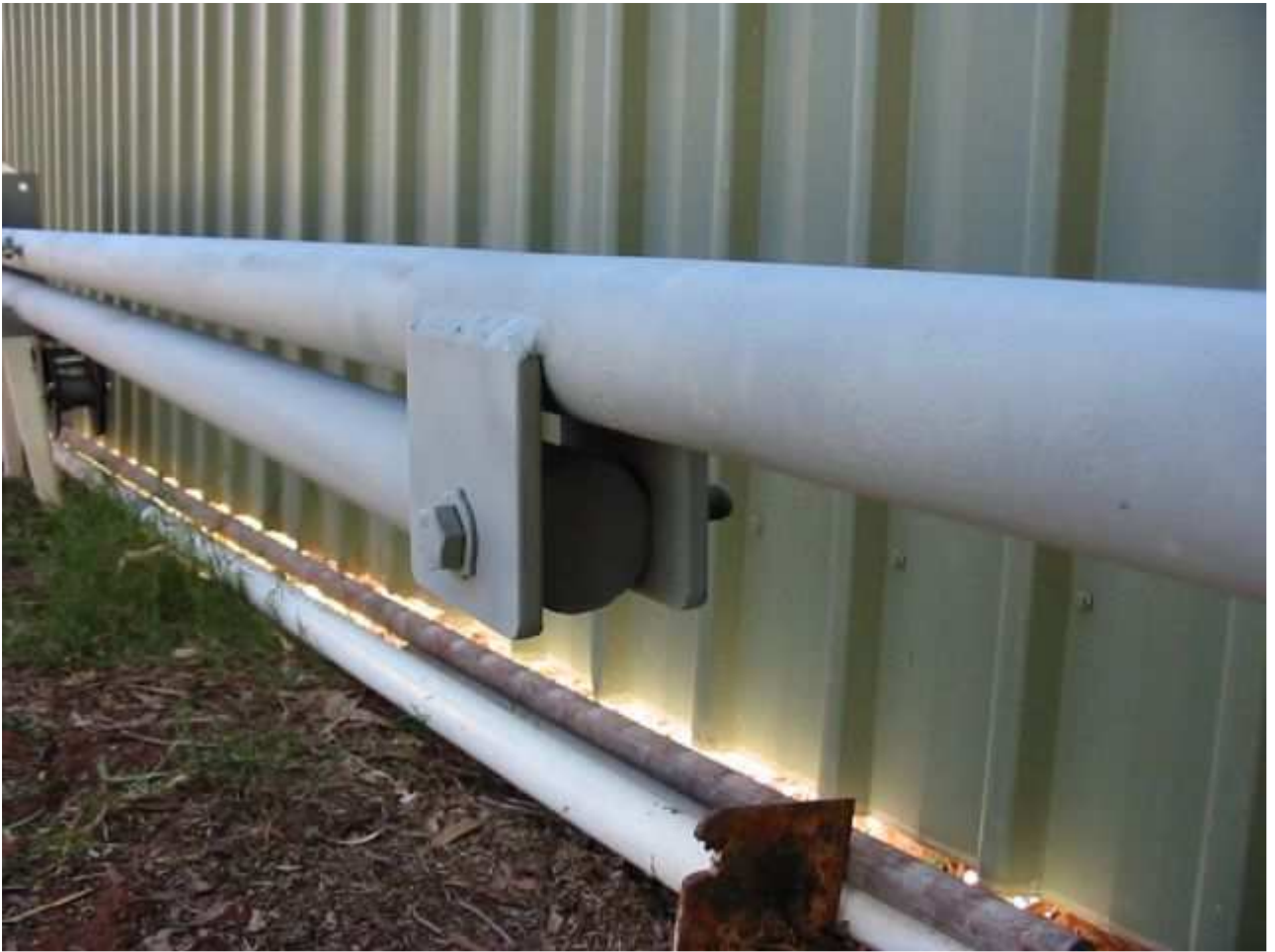
PIVOT POINT FOR TILTING OVER THIS SMALL TOWER.
