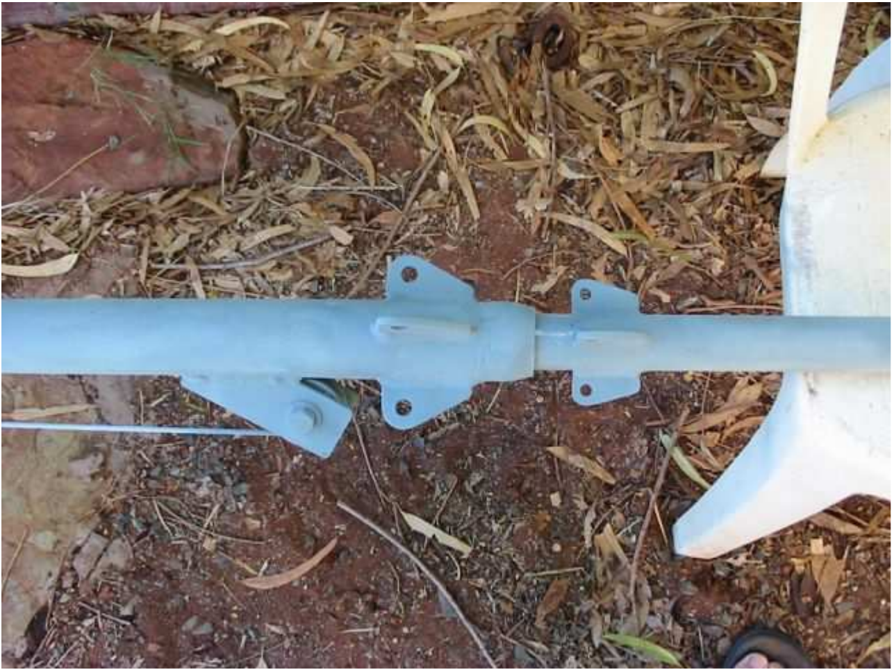
TOP PULLEY, OUTSIDE SECTION AND INSIDE SECTION. ALSO, MIDDLE AND TOP GUY WIRE POINTS.
